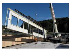
because of less weather delays and helps ensure building quality. For the on-site construction, because most of the building is already made, only the material really needed is transported which cuts down on emissions from transportation. Additionally there is generally less impact on the construction site area because less space is needed to store building materials also shorter construction time and easier construction
